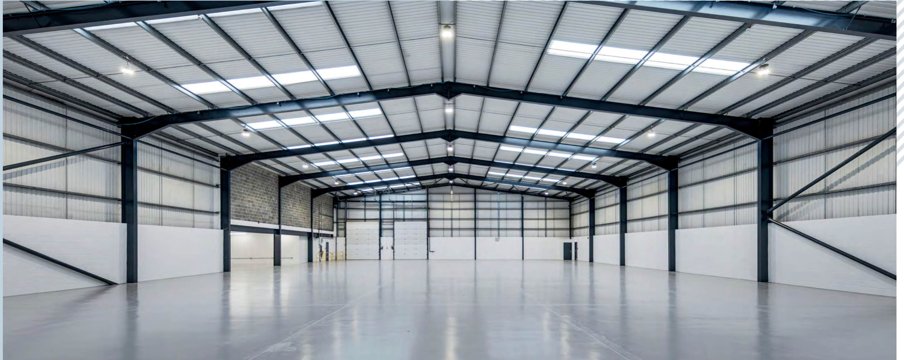
7.64m clear height & 2 electric loading doors
