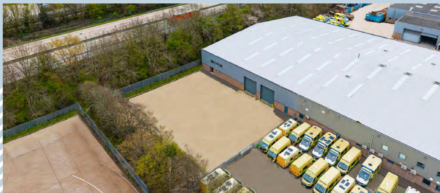
Newly refurbished spacious warehouse
