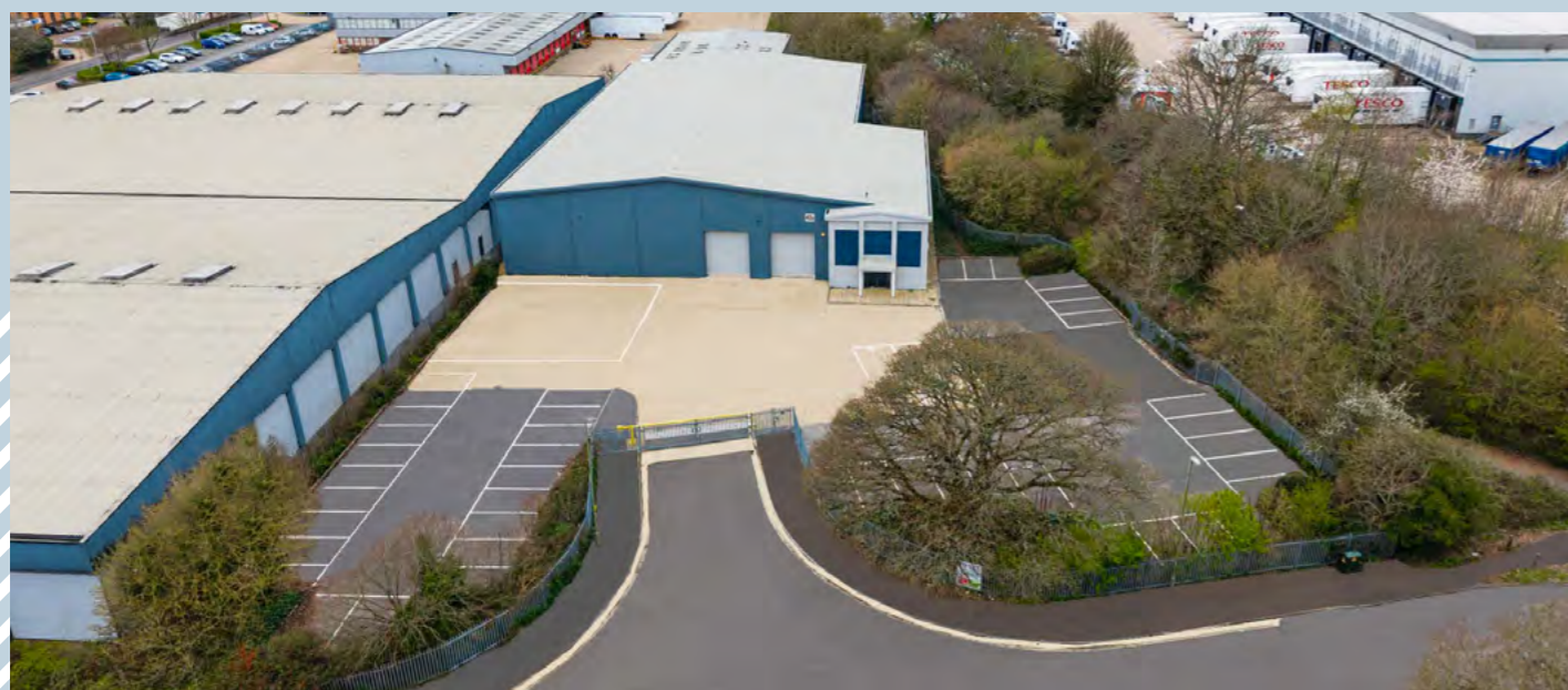
Spacious warehouse with roof lighting and secured yard
