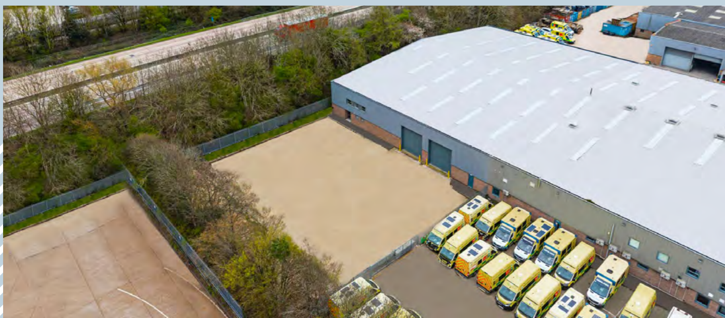
Newly refurbished spacious warehouse
