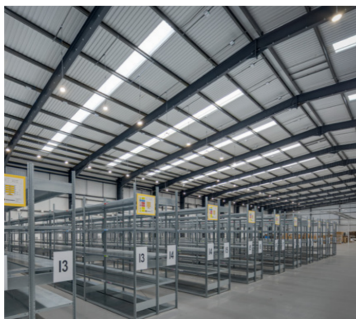
Warehouse fit-out includes low level racking, LED lighting, and warehouse W/Cs
