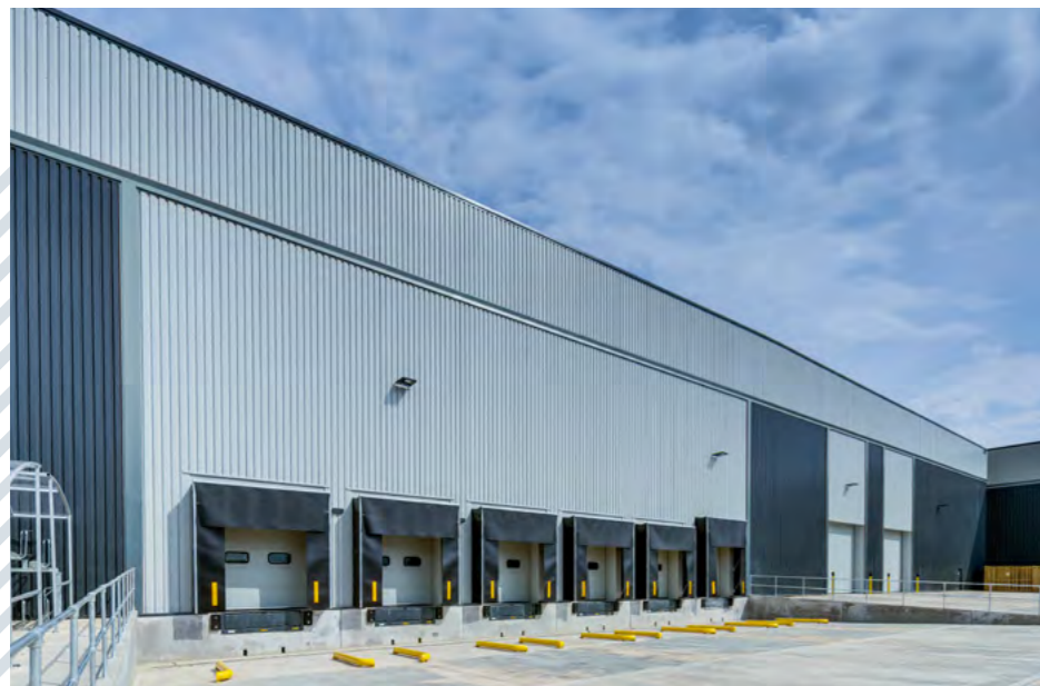
5 dock level doors & 1 euro dock level door
