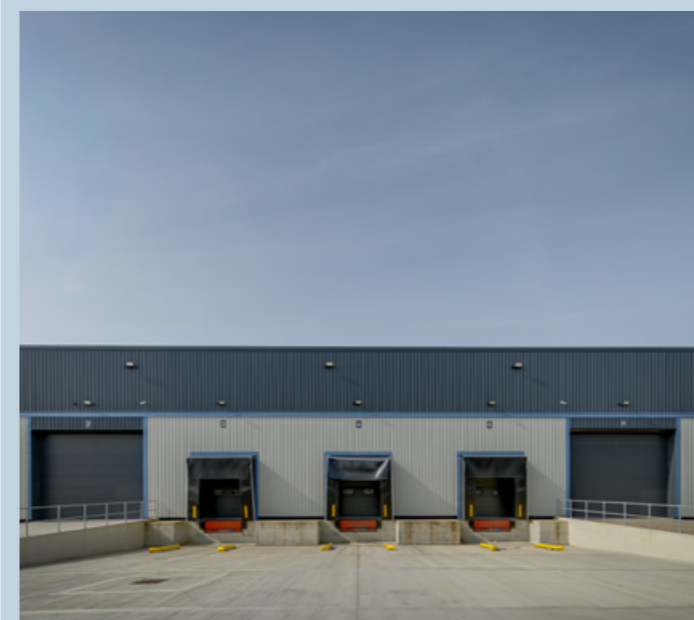
3 dock level doors & 3 level access doors
