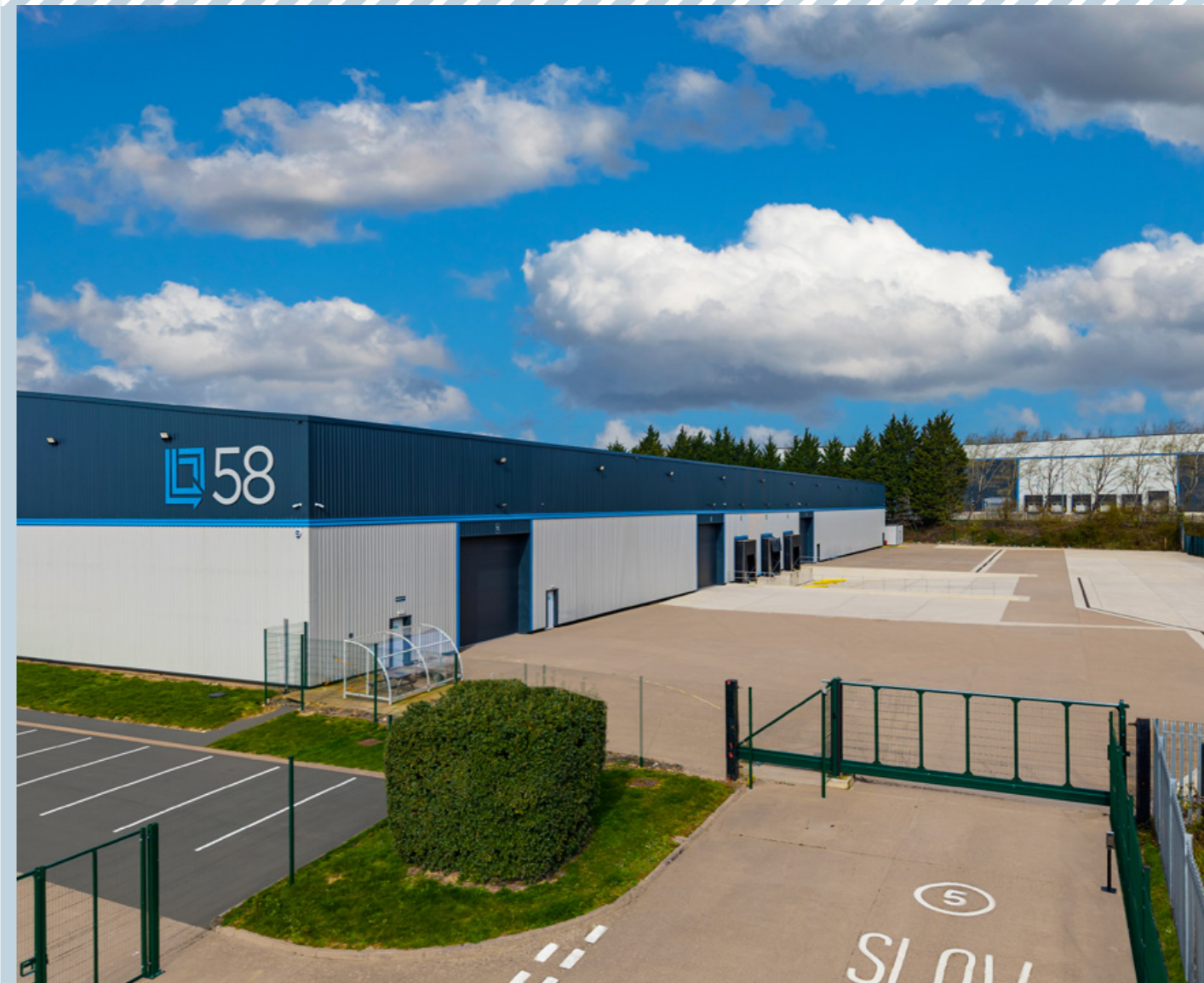
40m Secured Yard, Floor Loading 50 KN/M 2
